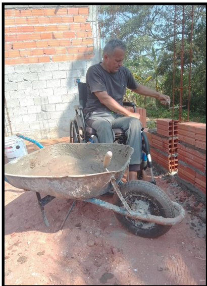
Working on the house
