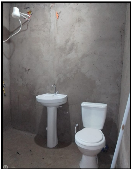
An Inside bathroom
