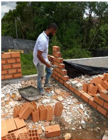
Starting a new house
