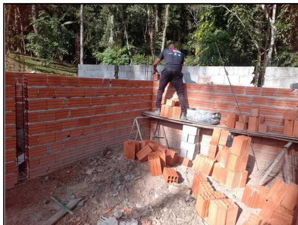
Up go the walls
