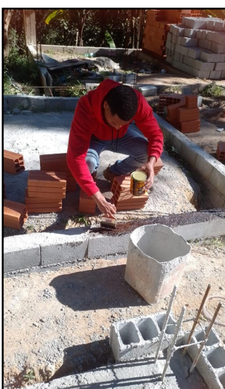
Setting the perimeter
