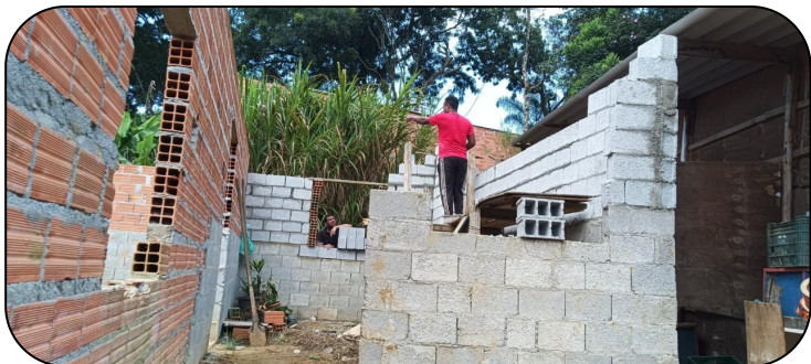
Walls going up
